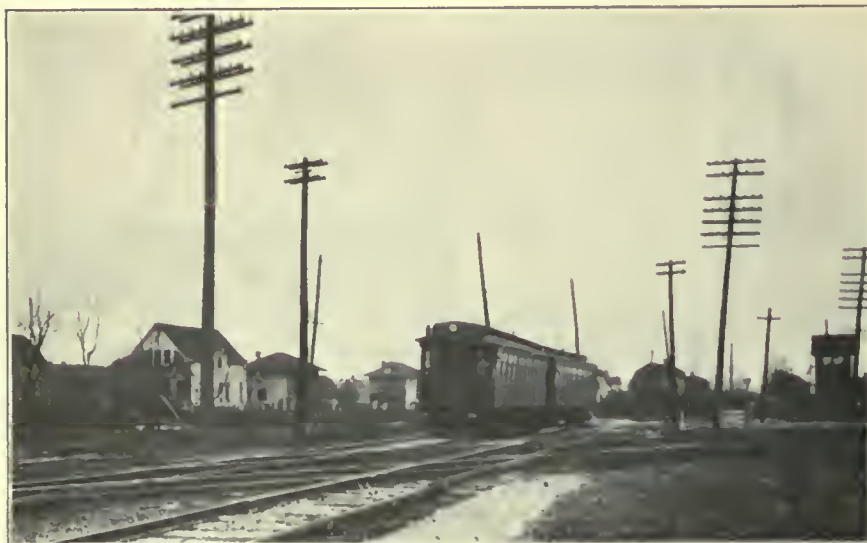
FIG. 252. GRADE CROSSINGS. Crossing of the Metropolitan "L" and the Baltimore & Ohio Chicago Terminal Railroad at Forest Park, Ill.
